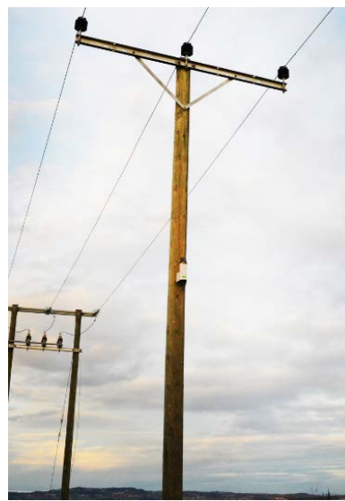
Pole Mounted Indicator
